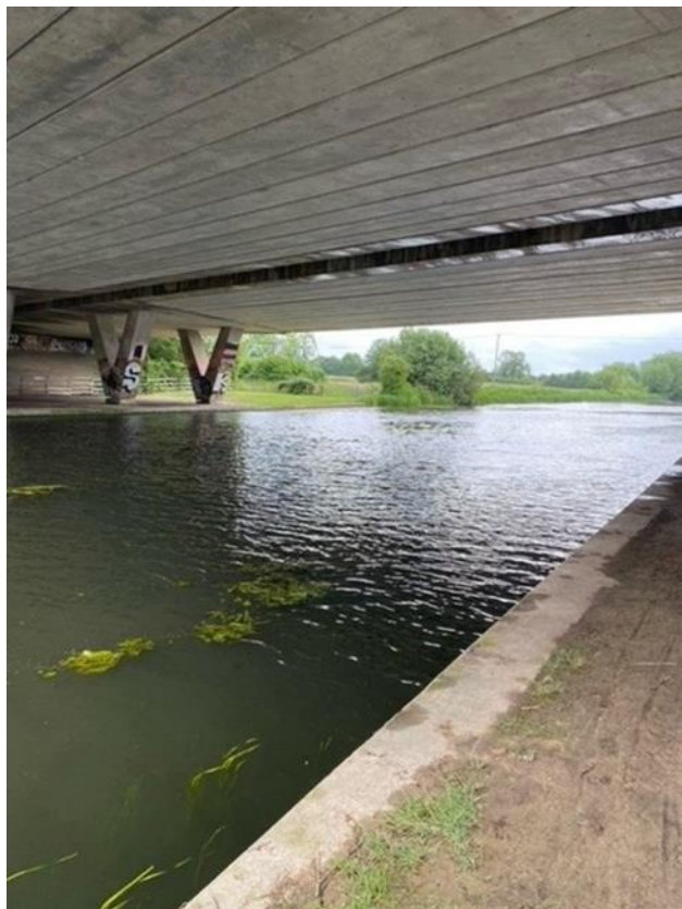
Figure 3.11: Example of bridge (module 2, upstream)
