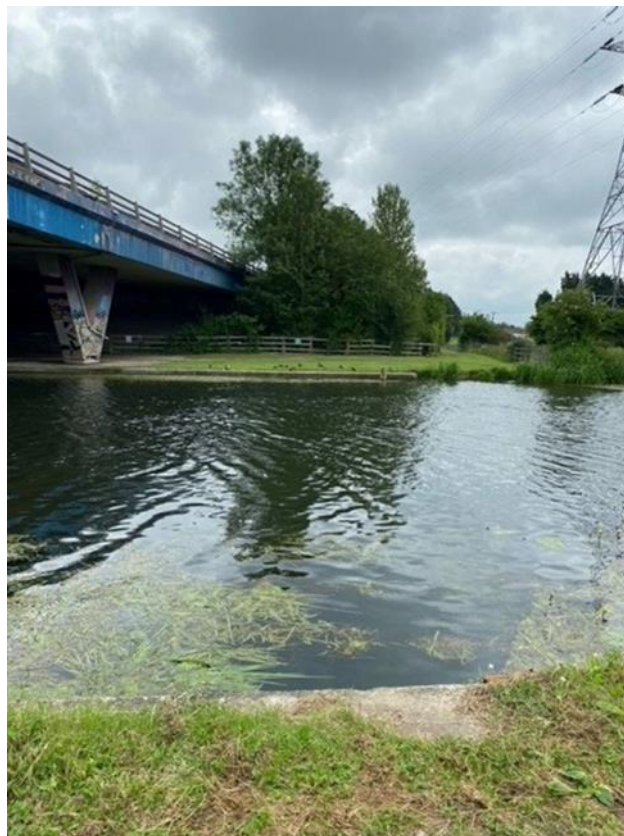
Figure 3.12: Channel aquatic morphotype richness with example of weed cutting (Module 1, cross section)
