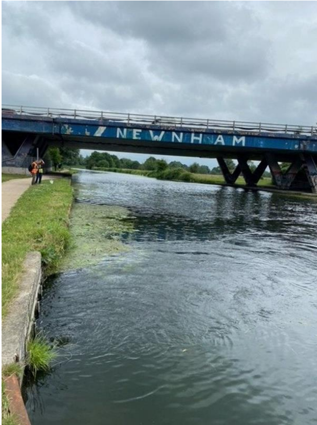
Figure 3.5: Bank top managed ground cover example and outfall (Module 1, downstream)
