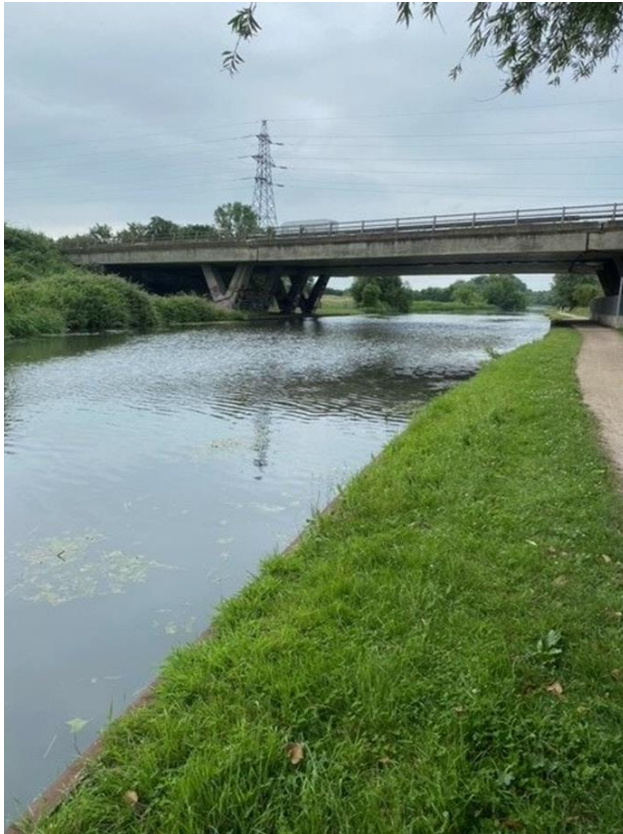
Figure 3.6: Bank face artificial profile extent example (Module 3, upstream)
